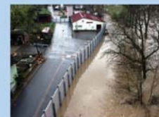
Overview of the same mobile protector like in picture 5. Flood event in 2002 (Kochendorf).
